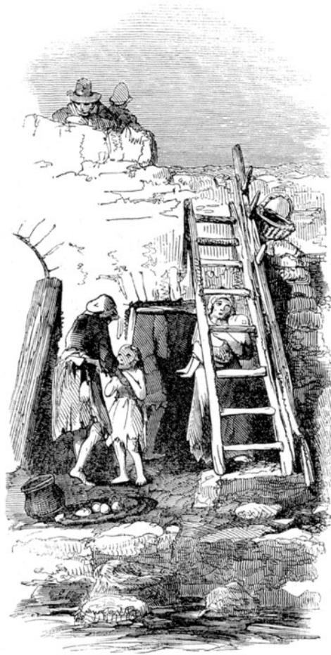
Judy O'Donnell's "home" under the bridge at Donnbeg, Clare, Ireland (1849).
